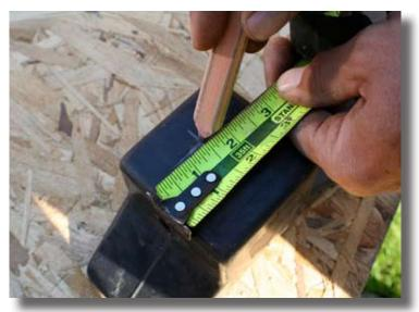
Take the Boat Bow and measure and mark the halfway point. The Bow featured is 3" wide at the base so the mark is at 1.5".
