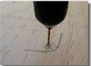
Using your Small Drill Bit (which matches the size of the Self-taping screws), drill a pilot hole on your four marks.
